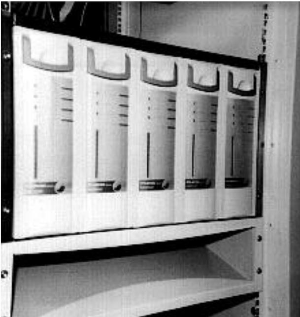
**Fig 5.** Magazine of 25A SMRs in a 19 inch rack.
